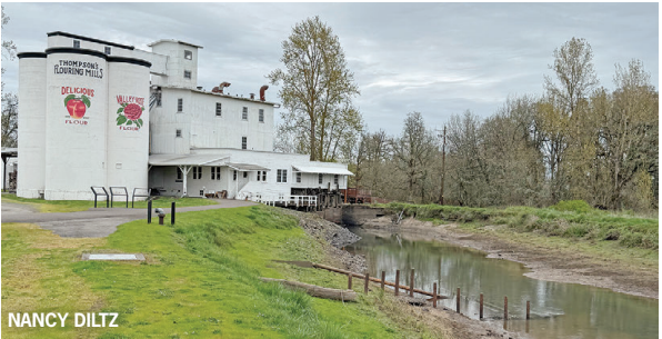
Thompson’s Mill, Shedd, Oregon
