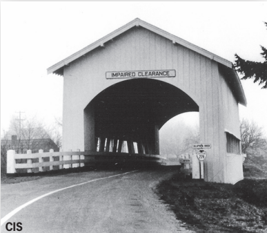
Built in 1932, the Crawfordsville Covered Bridge replaced earlier crossings over the Calapoovia River and remains a local landmark.
