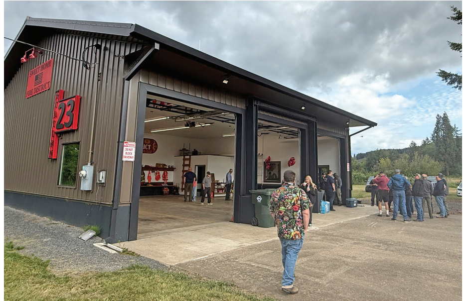
Community members, firefighters, and fire district leaders gather at Station 23 during the June 9 open house. The event welcomed residents to tour the renovated facility and reconnect with volunteers past and present.
