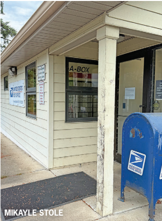
Crawfordsville's post office sits closed for repairs in late May. Postal customers are currently being served through the Brownsville Post Office while work is completed on the Crawfordsville facility
