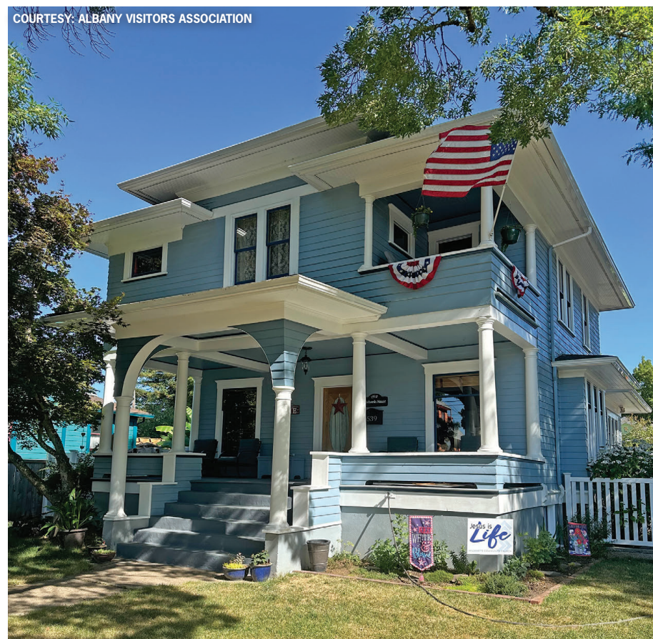
The William Richards House, built around 1910 at 539 Third Ave. SE in Albany's historic Hackleman District, is an excellent example of the American Foursquare architectural style. Named for its original owner, the home is a historic contributing property within Albany's National Register Historic Districts. The house was one of the featured homes on last year's Summer Historic Interior Home Tour, giving visitors a rare opportunity to explore its beautifully preserved interior.
