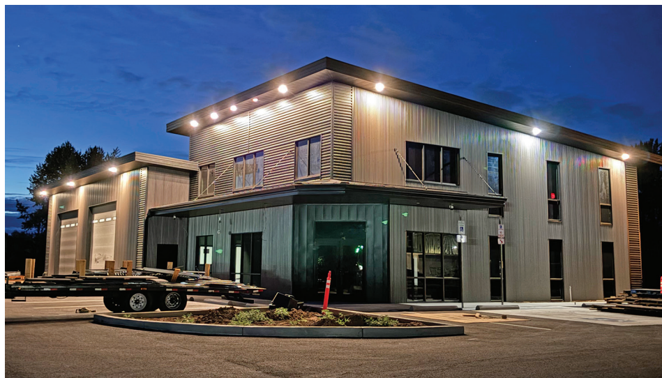
Exterior lights illuminate Pure Energy's new Albany facility as construction nears completion.
