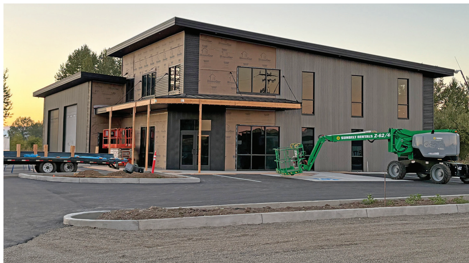
Pure Energy's new Albany facility takes shape as the solar installation company expands its presence in the Willamette Valley.
