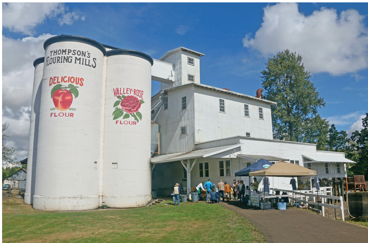
Visitors gather at historic Thompson's Mills near Shedd for a cider pressing event. The mill, built in 1858, preserves a piece of the Willamette Valley's agricultural history.
