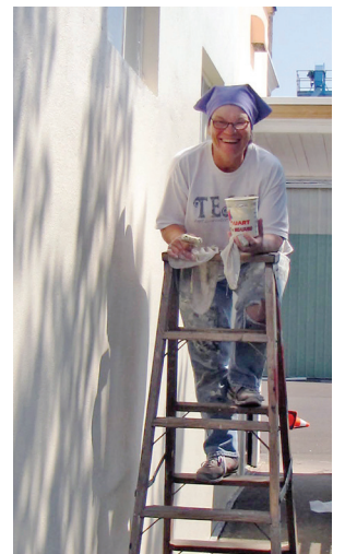
TJ Gillson works on painting the exterior of the historic library during the community-led restoration project.
